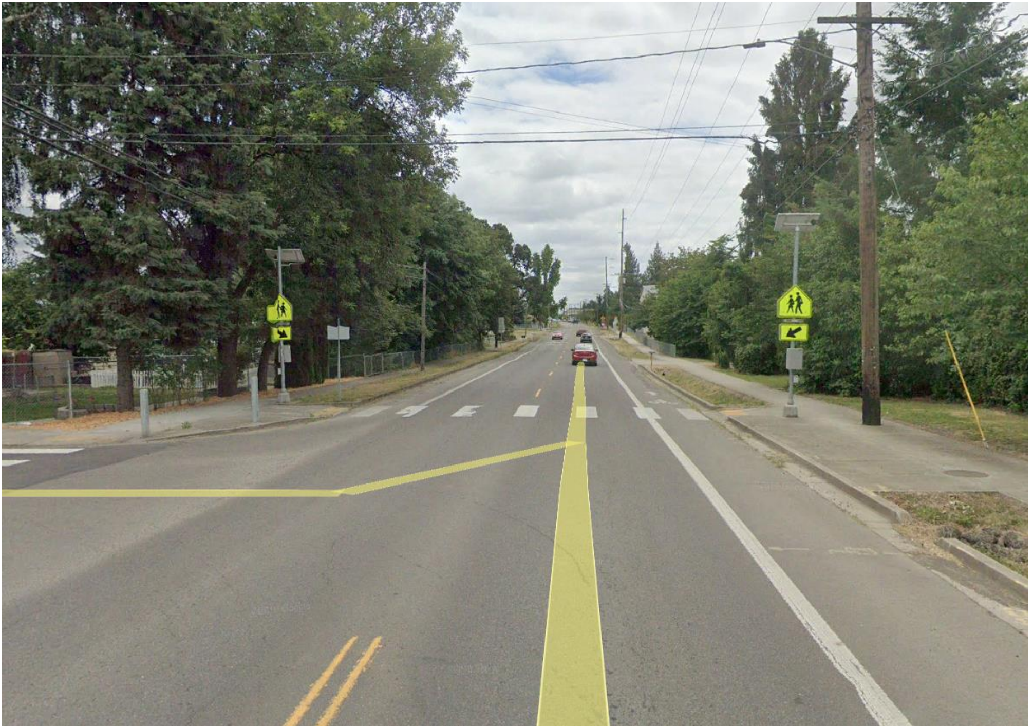
RRFB (Rectangular Rapid Flashing Beacon) Example City of Amity – Intersection of Rice Lane and OR99 (Trade Street)
