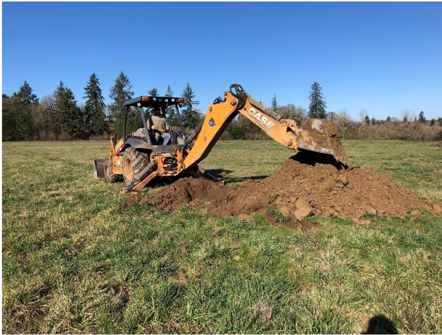
Test Pit TP-8
