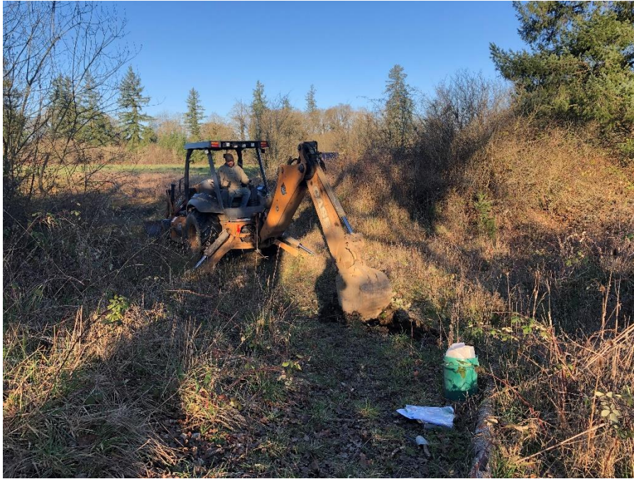
Test Pit TP-1
