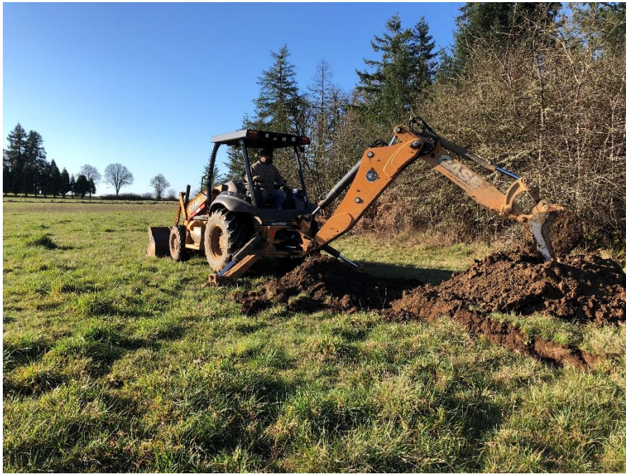
Test Pit TP-4
