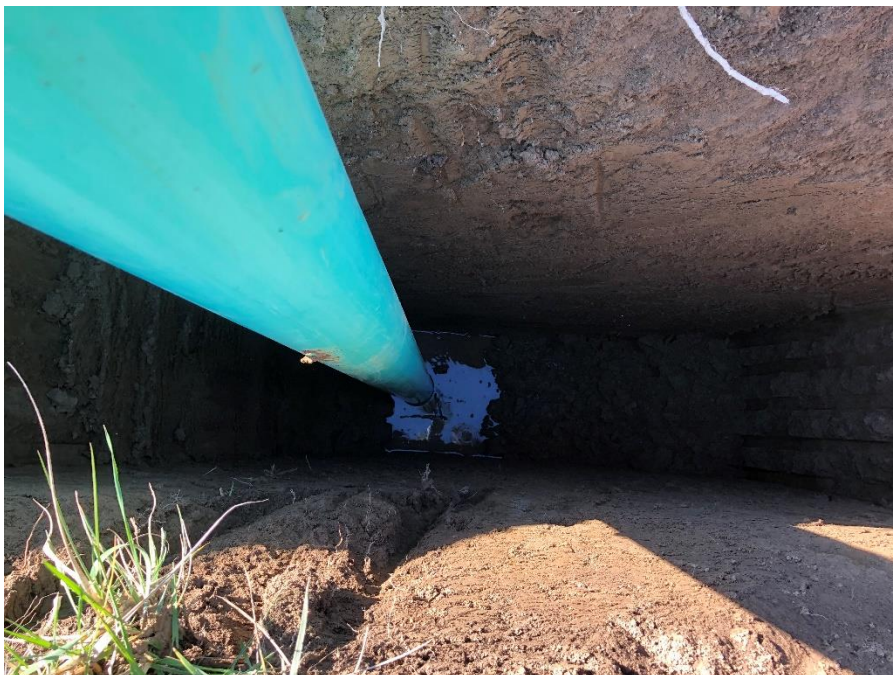
Test Pit TP-3
