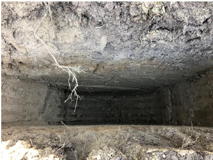
Test Pit TP-5
