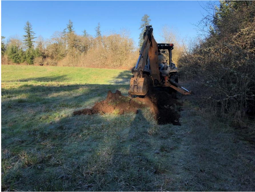
Test Pit TP-2
