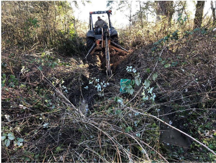
Test Pit TP-5
