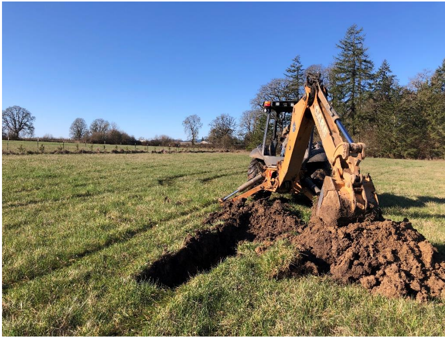
Test Pit TP-7
