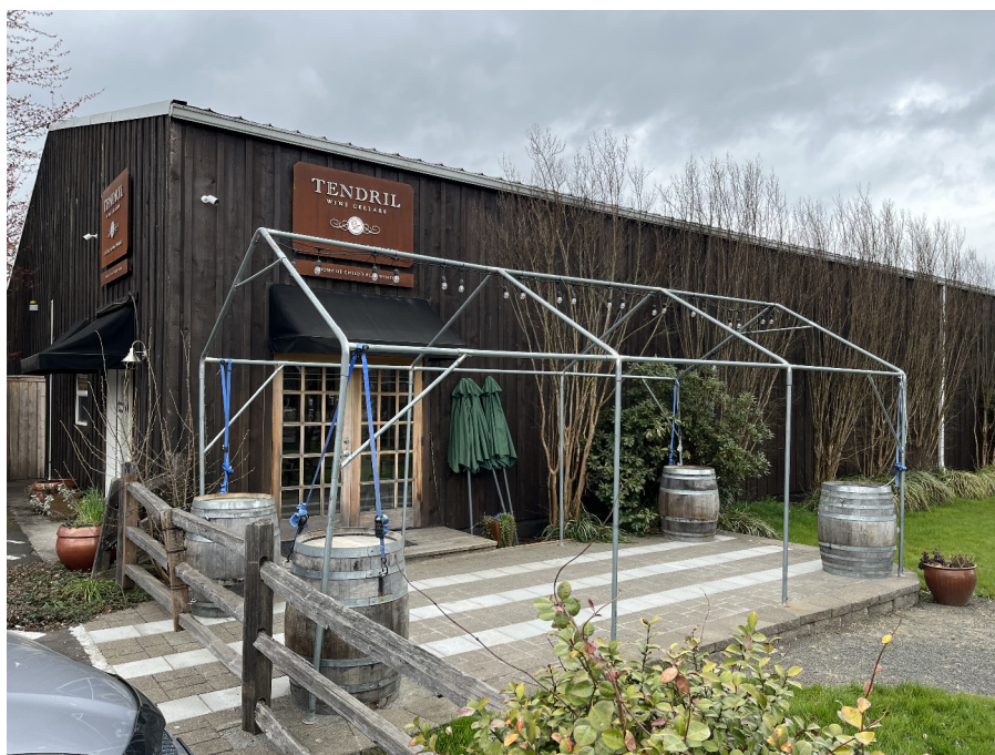
SOUTHEAST CORNER OF THE BUILDING
