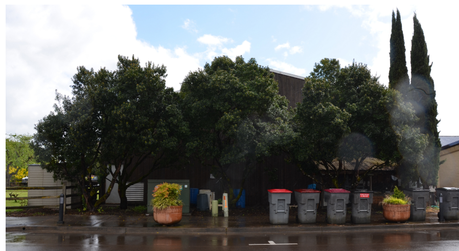
NORTH SIDE OF THE BUILDING
