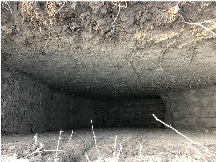
Test Pit TP-2
