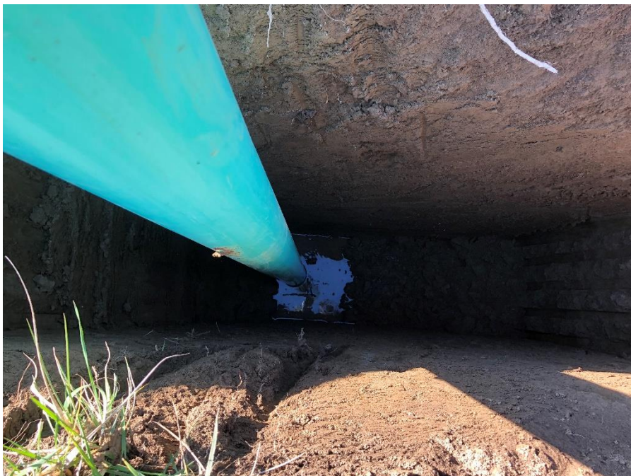
Test Pit TP-3
