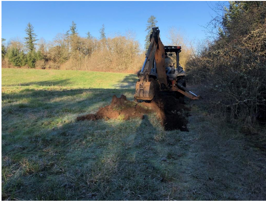
Test Pit TP-2
