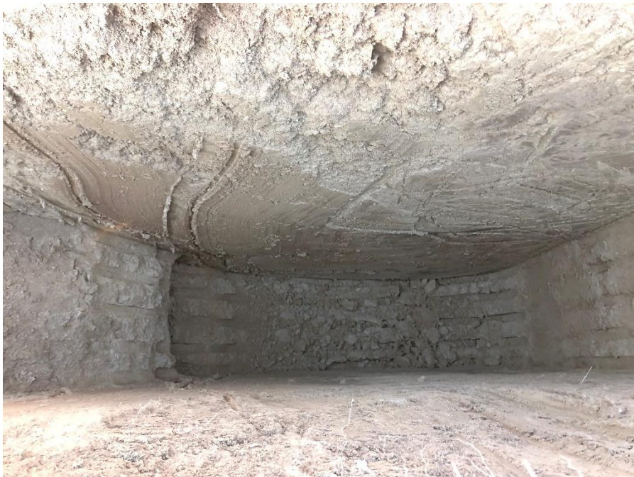
Test Pit TP-4
