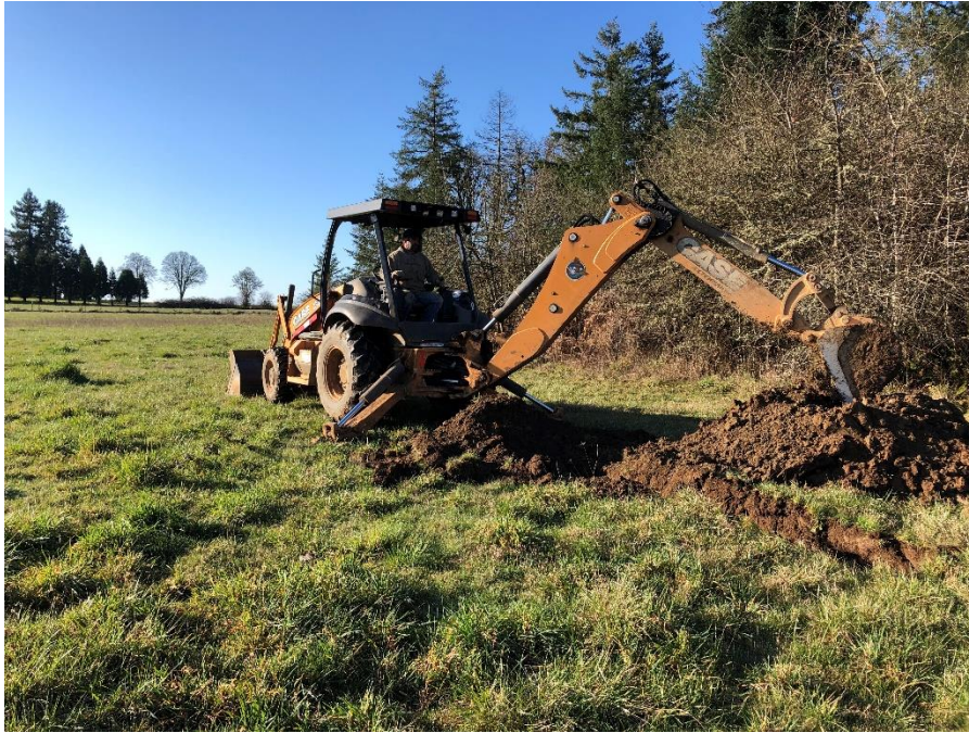
Test Pit TP-4
