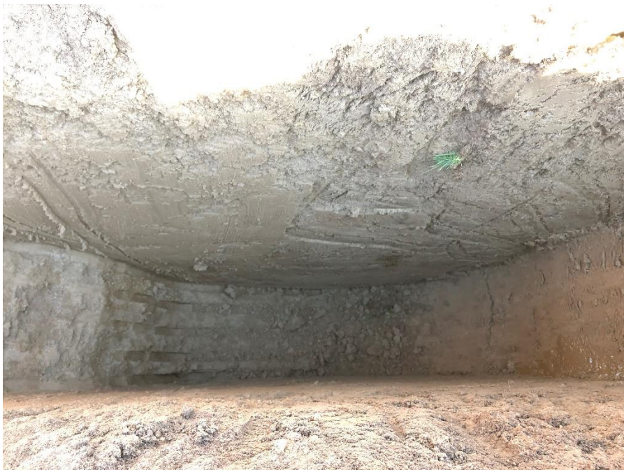
Test Pit TP-8
