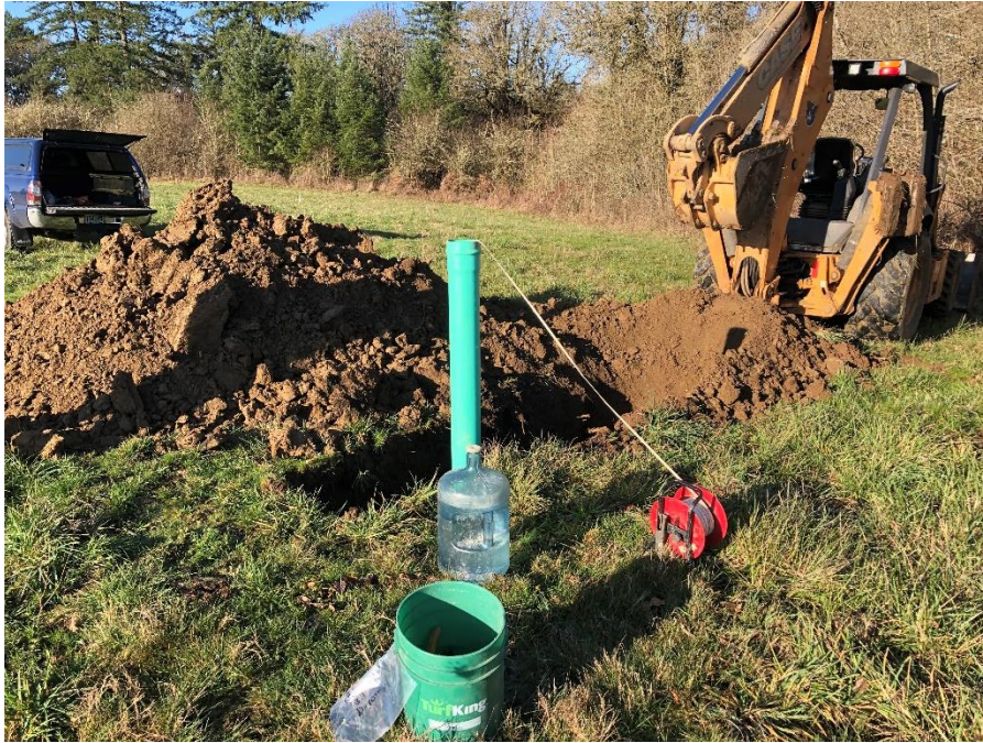
Test Pit TP-3 With Infiltration Testing at -10 Feet bgs
