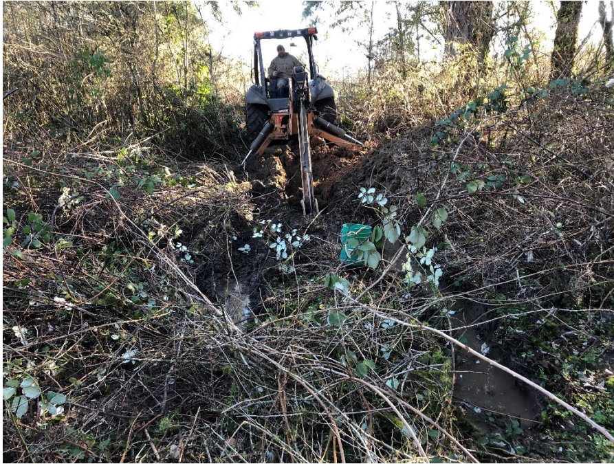
Test Pit TP-5
