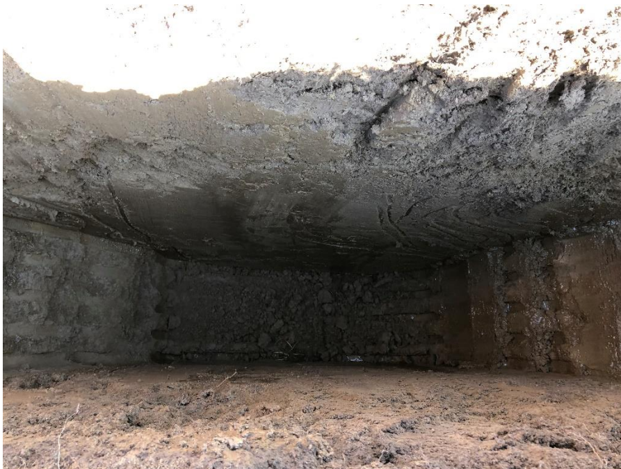
Test Pit TP-7
