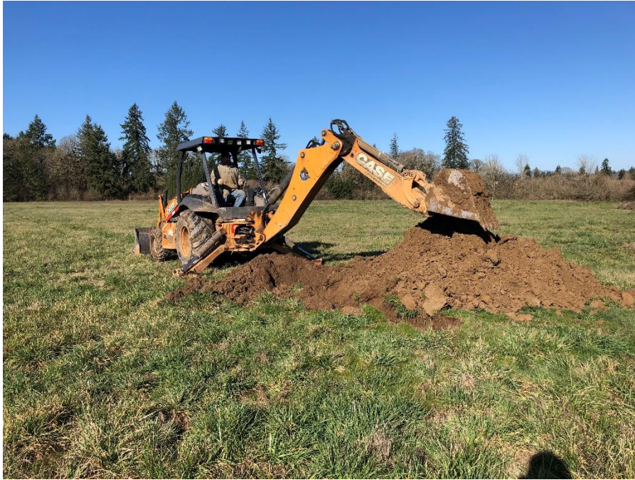
Test Pit TP-8
