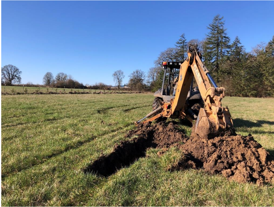
Test Pit TP-7
