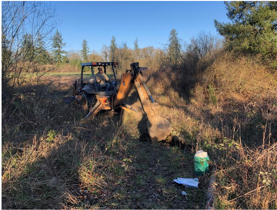
Test Pit TP-1
