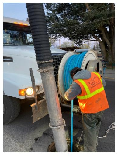
➤ On the construction side of the sewer, the building project on Washington St. the Flaneur building is required to install a new sewer main on Washington from 1st to 2nd ST. This is approximately 225′ of new 8″ pipe and two new person holes & connection of all existing laterals to the new pipe.
