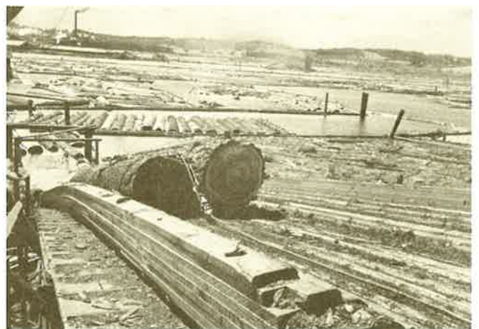
Log ramp used to bring logs from the lake to the Carlton Mfg. mill. Across lake is the L.H.L. mill in operation.
