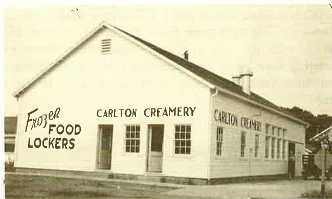
Bill and Opal McGhie opened the Carlton Creamery and Lockers in this new building in 1940.
