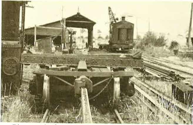
Big steam loader poised in front of Carlton roundhouse.
