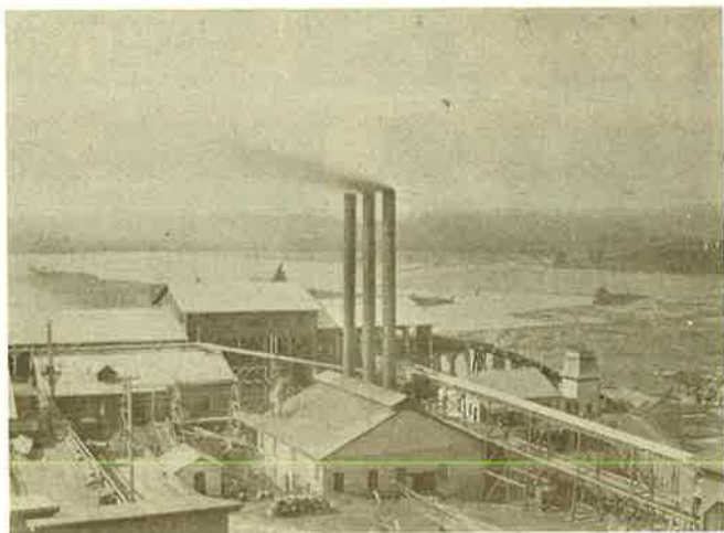
Consolidated mill located on the Carlton lake. The largest mill to operate in this region. It burned about 1914.
