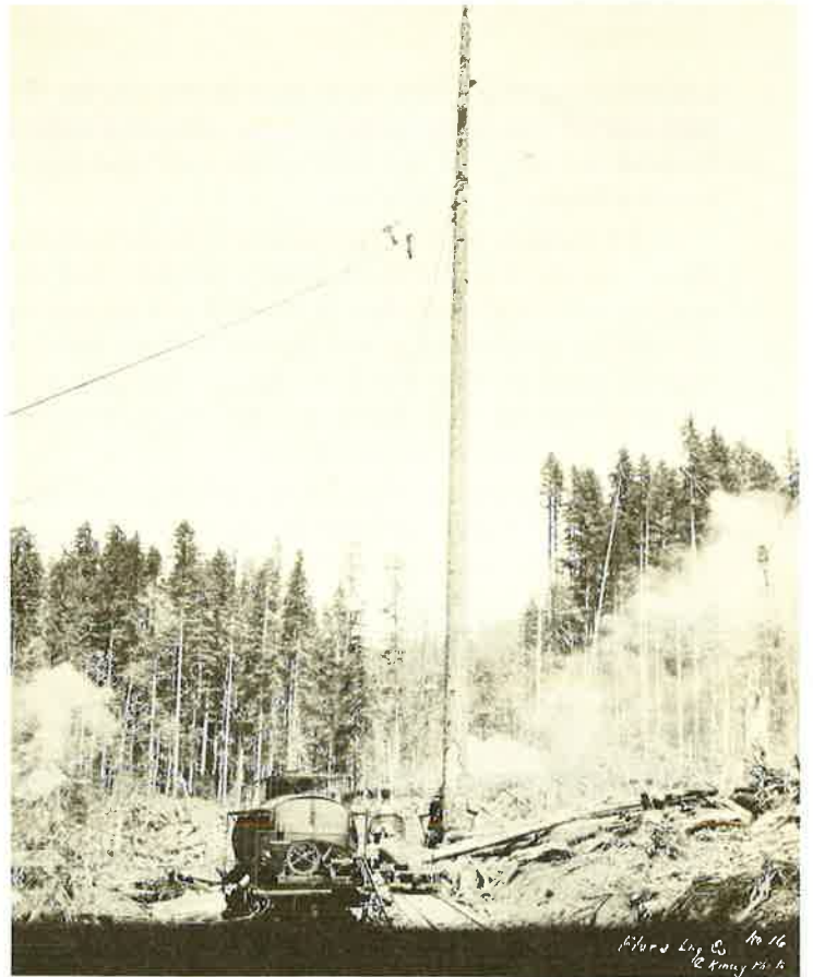
Flora loading donkey with high rigger still atop the spar pole doing what only high riggers and circus people might do.
