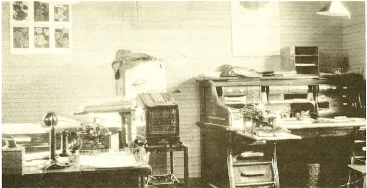
Telephone typical for office use in 1936 in Carlton Nursery.
