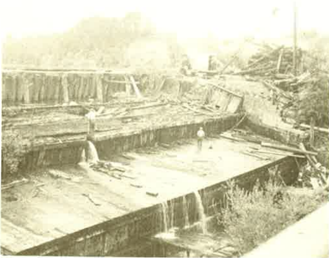
Crew from the L.H.L. mill start repair of the dam in 1951.
