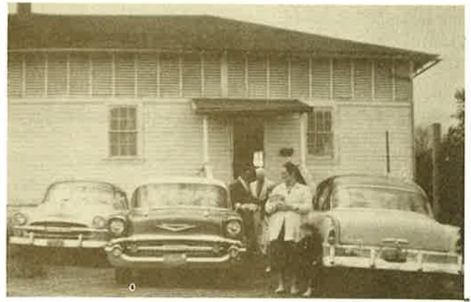
Old Carlton School Annex which was later used by the Assembly of God Church in 1948.
