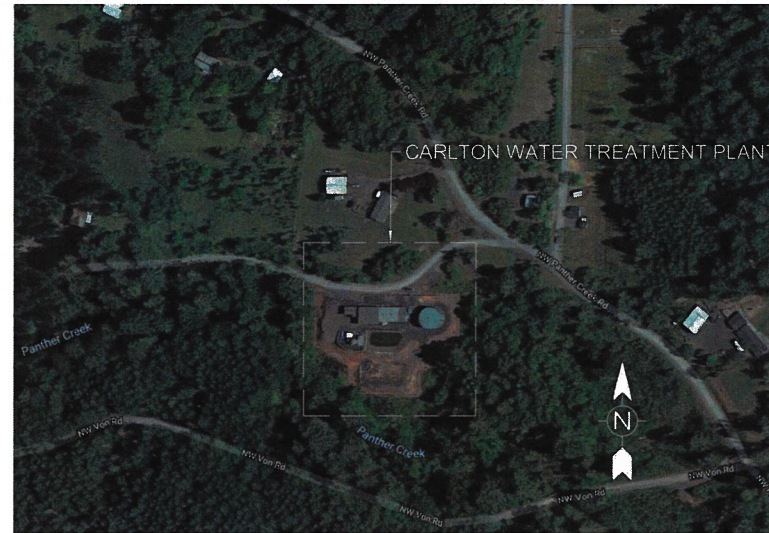
PROJECT SITE - WATER TREATMENT PLANT
